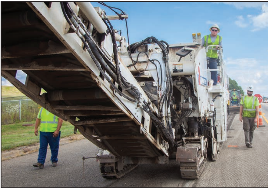
With Roadtec's focus on high-powered, balanced production, Welfle crews are routinely able to mill 120-140 feet/min., and 25,000 yds. or 5,000 tons/day. (Pictured: Roadtec RX500 on Rt. 62, east of Alliance, OH, with Foreman Ken Smith and crew.)
