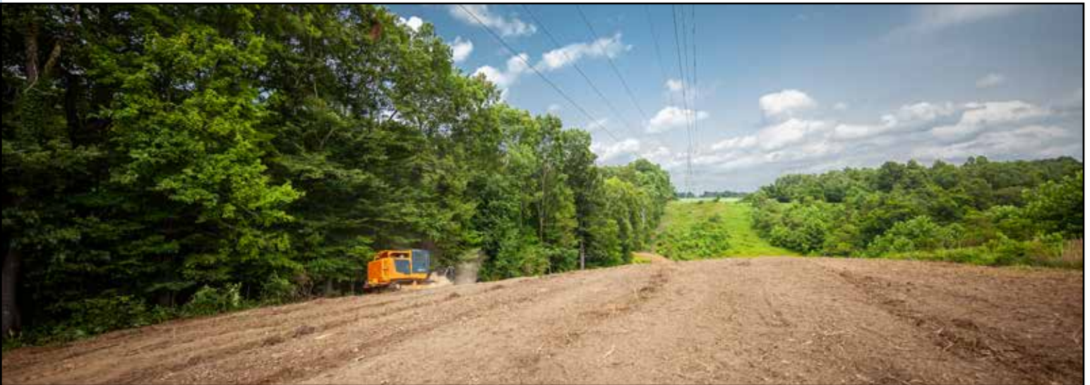
Jerrod Watts has an entire career of land clearing experience. Watts is pictured above in a CMI C400 clearing for a 12-mile, 138 kV transmission line rebuild just outside Philo, Ohio.
