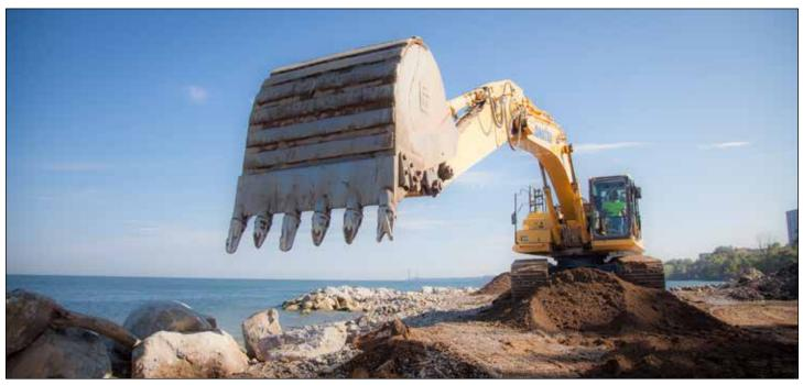
Haynes' Komatsu PC360i excavator played a key role in the grading and excavating of 10,000 cu. yds. of earth and placing 35,000 tons of armor rock revetment as part of the Euclid Shores Improvement Project for the City of Euclid, Ohio. The project also entailed utility pipe work and a half-mile, walking trail.
