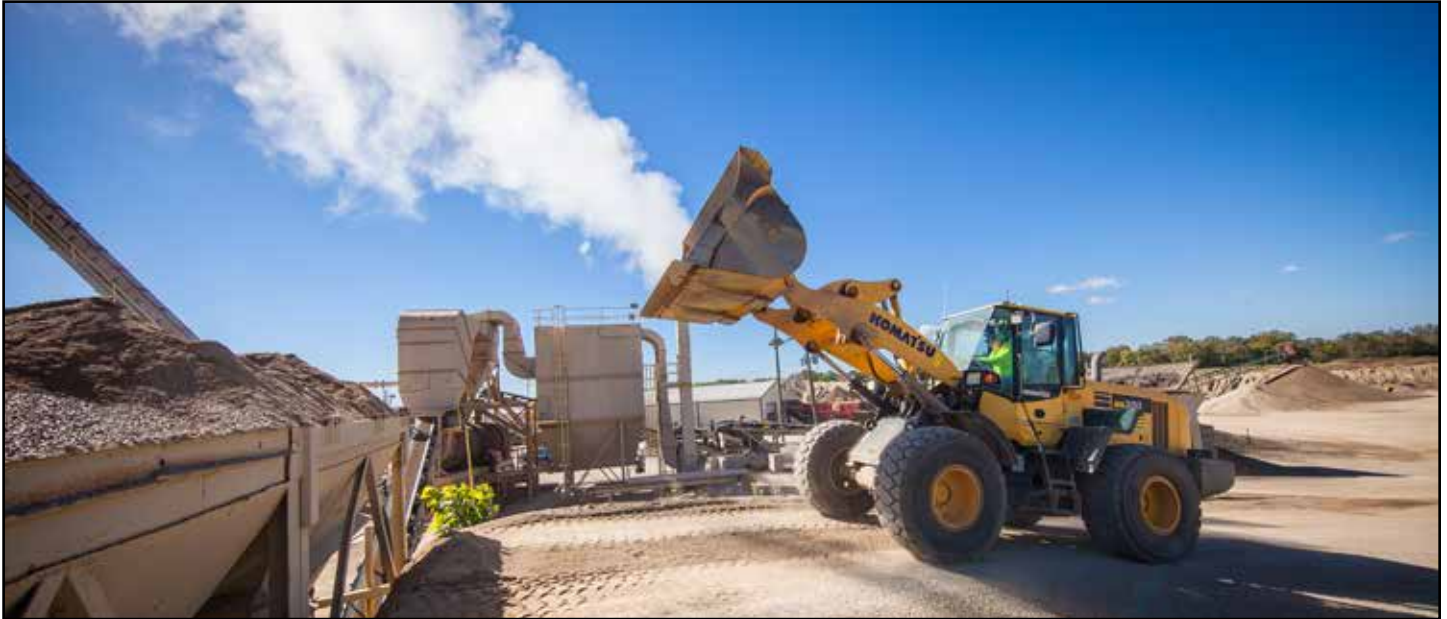
The G&J Paving plant produces around 70,000 tons/year, with 90% of that production being channelled internally, onto company projects. Recent maintenance upgrades mean the plant can now run throughout the winter, as long as the materials remain unfrozen.
