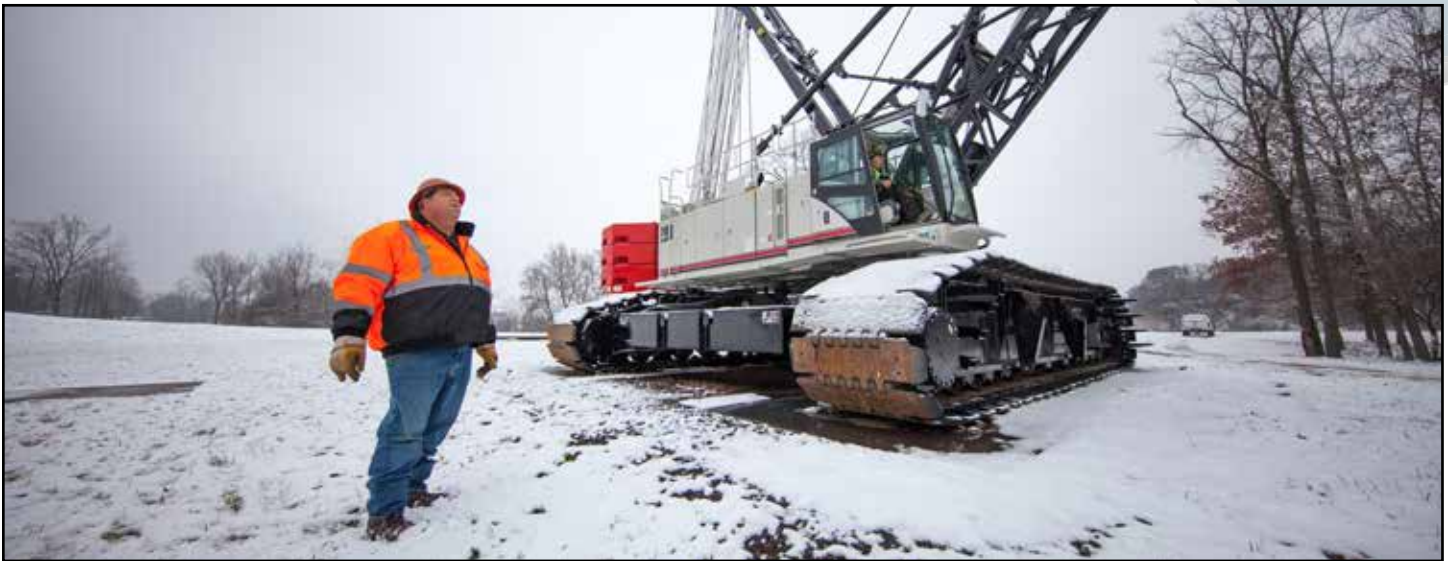
Hoisting and Rigging Instructor John Haberkorn brings over 25 years of lifting experience to the JATF program. Today, he takes great pride in contributing to a program that nurtures the next generation of lifting professionals.
